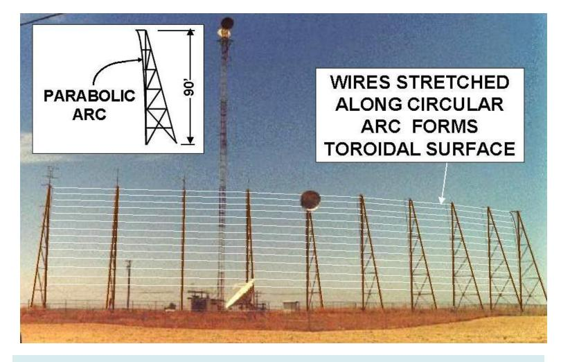
Above is an image of a halfbolic antenna that had been installed in California in the late 1960's. The photo shows the back side of the antenna. The parabolic antenna near the center of the tower was most likely a microwave link back to the city.
