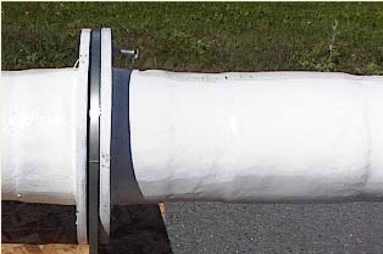
Here is a close up of the radome flange area. The fiberglass near the flanges has been thickened with extra layers of material to prevent cracking. The flanges are also thicker than the main body of the radome. An aluminum radome stop between the flanges is part of the support system of the antenna.
