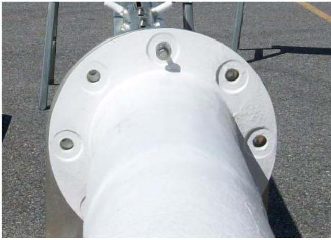
The picture to the left shows the Radome flange on a side mounted UHF slot antenna. The flange area is thickened up to provide superior strength. The first 6 inches of the radome itself has extra layers of Fiberglass to eliminate cracking.
